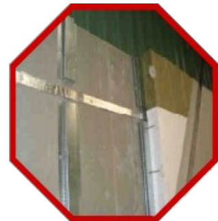
FF102/25 Ventilated Fire Barrier installed behind cladding system
