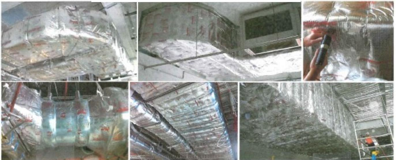
For Fire Protection from fire outside the duct
